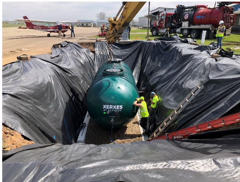
1: 8,000 Jet Fuel Tank Install
